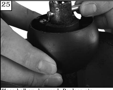
25 Place ball on downrod. Replace pin removed earlier and pull ball up so that the pin fits in the notches in the ball.
